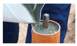
The Kebu sleeve tube filling compound is a permanently plastic compound based on technical petrolatum. With the compound you can fill cavities between the core tube and the rods on gates valves in transport and distribution networks.
